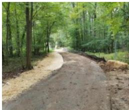
As Bolin Creek Trail construction resumes, extending the trail segment from underneath the Martin Luther King Jr Blvd bridge up to the existing trail, the contractor will also begin remediating the lower portion of the Police Station property. Remediation will include the removal of soils that contain coal combustion products, as well as the addition of “super” silt fencing and hydroseeding to control erosion along the embankment.
