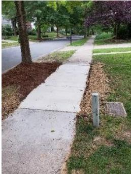
Over the past few months, the Construction Division of Public Works completed repairs on 585 linear feet of sidewalk at 35 different locations in Southern Village. Construction staff fixed tripping hazards, such as those caused by tree roots creating an uneven walking surface.
