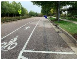
The Traffic Engineering Division hired a contractor to revise pavement markings on Meadowmont Lane from Sprunt Street to the end of the street. They added buffer bike lanes on both sides of Meadowmont Lane from Sprunt Street to Simerville Road; removed bike lanes and added curbside parking on the northside of Meadowmont Lane from Simerville Road to end of the street; and created a left-turn lane into Rashkis Elementary School.
