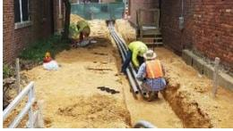
Downtown Alleyway Improvement Project: All demolition work in Post Office Alley is complete. The contractor has installed the conduit bank and soil has been delivered to bring the alley up-to-grade. Work on Varsity Alley will begin once work on Post Office Alley is complete. Both projects are on schedule and expected to be finished by September.
