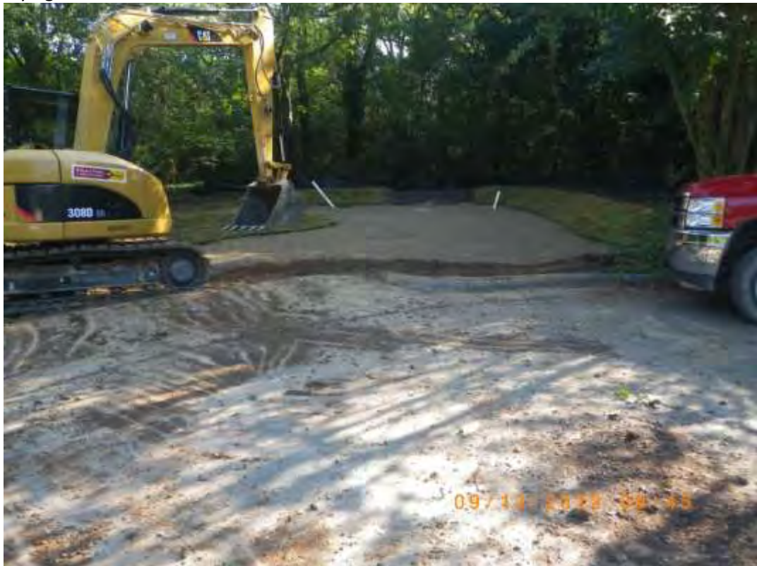
Filling in with soil media
