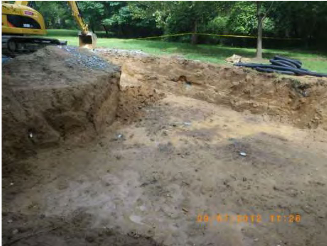
The basin is completely excavated
