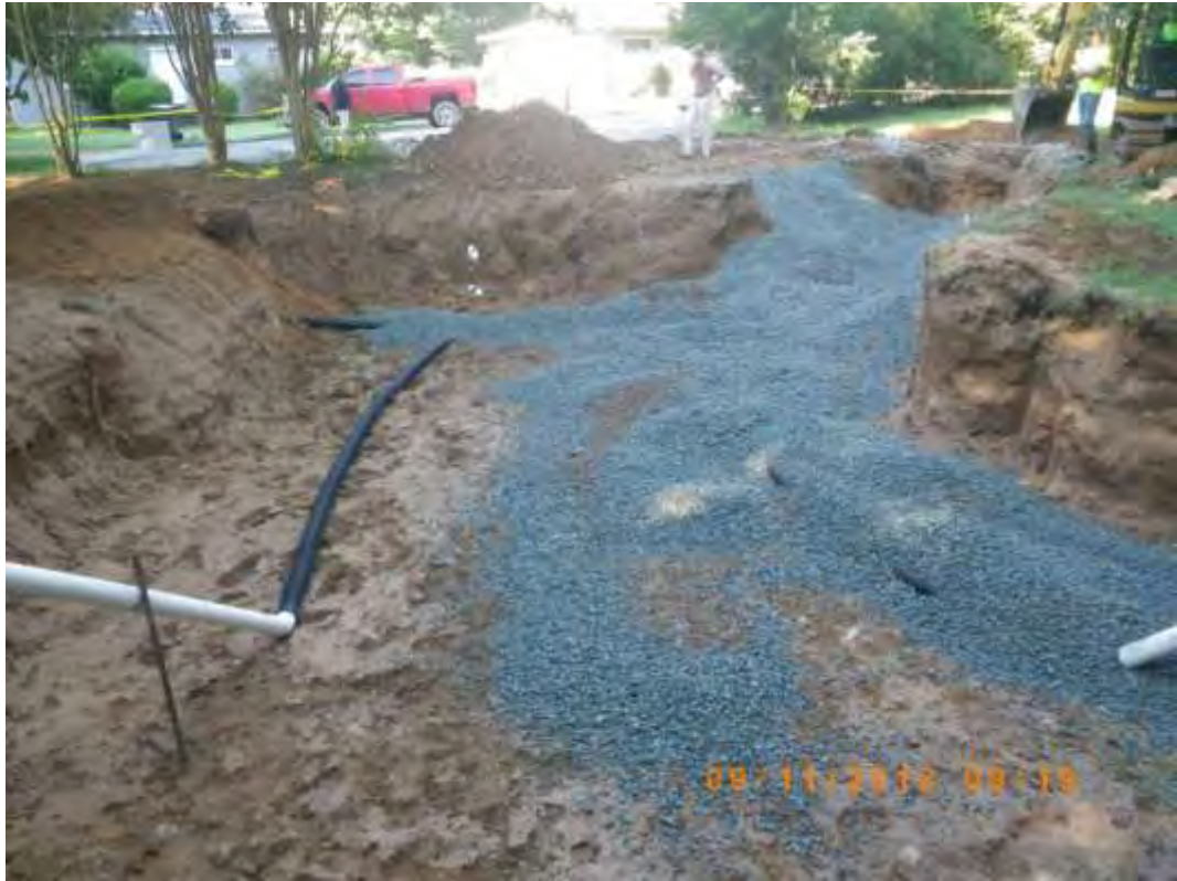
Laying the underdrains
