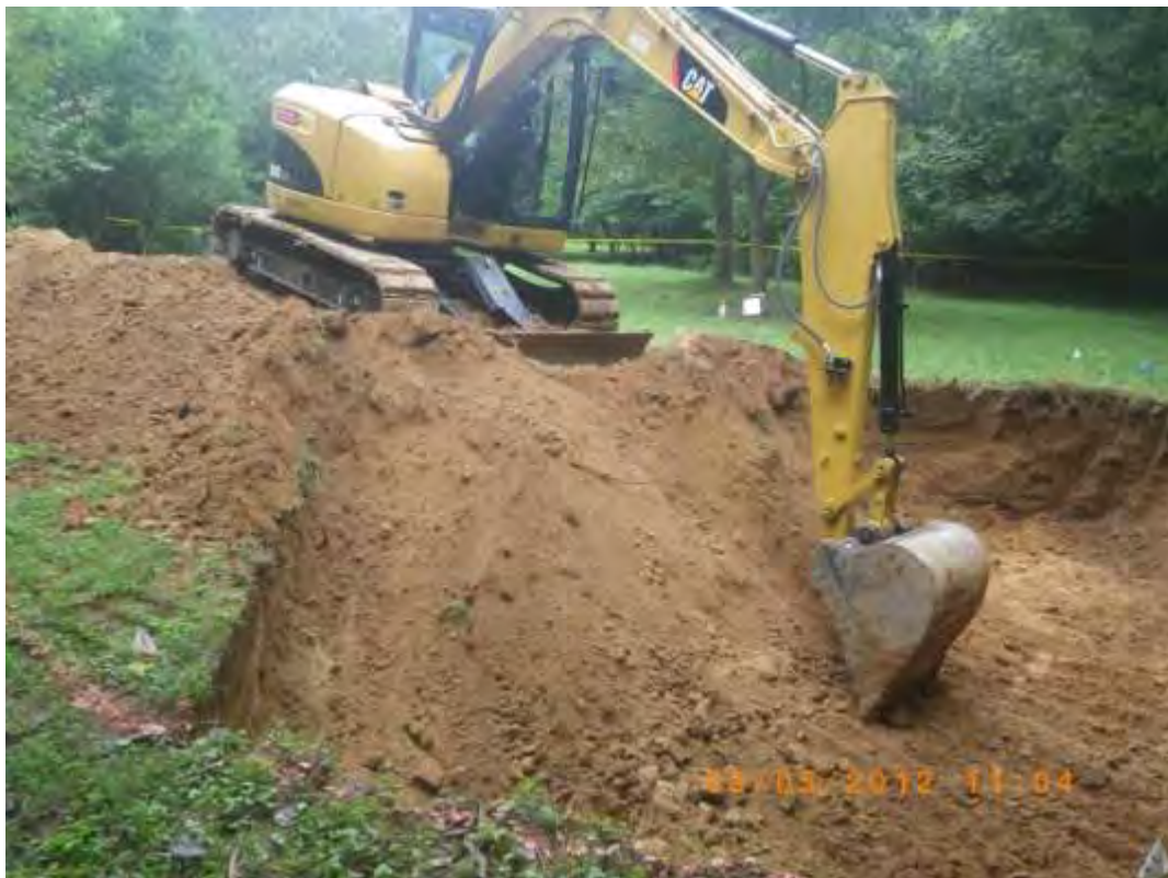
Starting to excavate the bioretention basin
